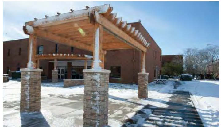
Student Center Renovations
