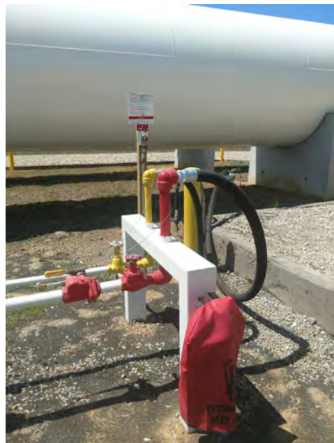
Bobtail Loading Bulkhead Example
