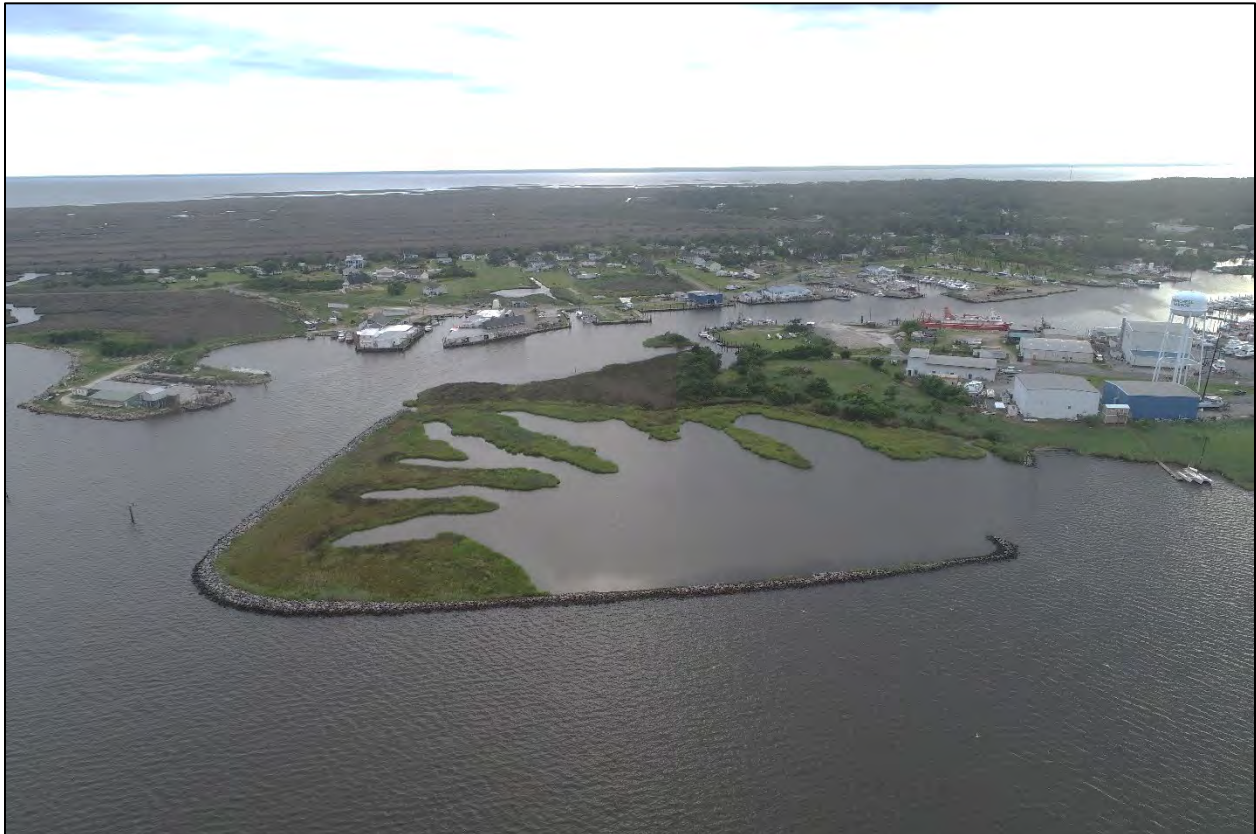
Figure 13. Drone image of the Wanchese Marsh Project taken July 2020.
