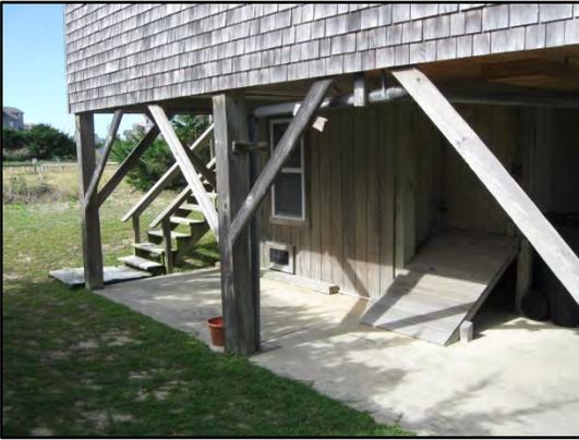
*Example of typical flood opening in enclosure.*
