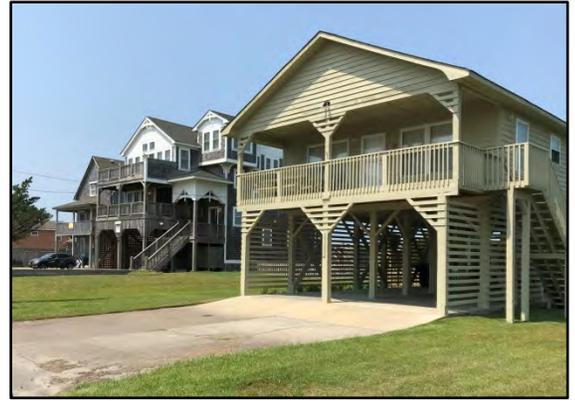
*Examples of structures in Waves village. Majority of homes are on piling foundations, many with ground floor enclosures for parking, access and storage.*
