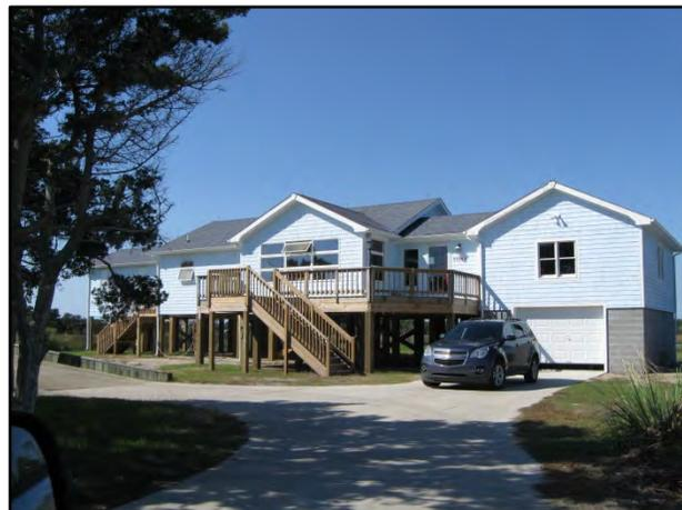
**Repetitive Loss Area H-10** is located within the AE flood zone. Multiple ponds are located within and a creek runs adjacent to the repetitive loss area. The area is residential with the majority of properties being Pre-FIRM and having piling and crawl space foundation styles. Flooding occurs from over the bank flooding from adjacent and nearby ponds and canals.
