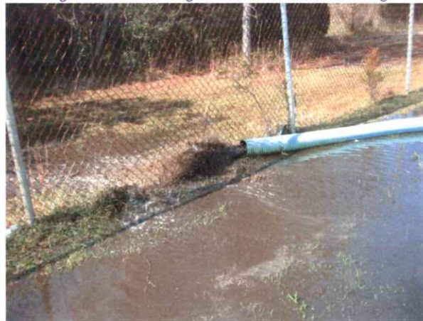
Figure 3-1 - Drainage from Clearwell Cleaning
