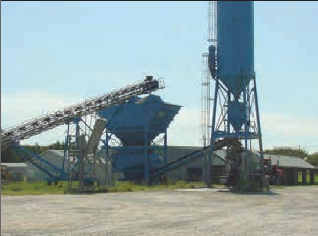
Concrete manufacturing plant components
