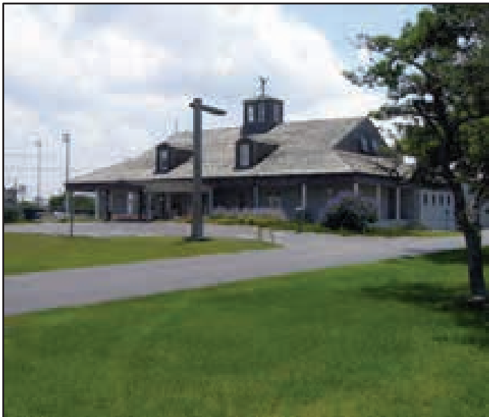
Dare County Reverse Osmosis Plant in Kill Devil Hills
