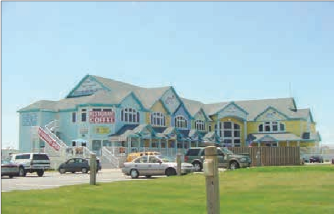
Large multi-unit commercial structure
