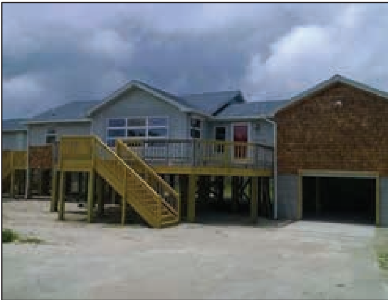
Example of a building that was elevated to mitigate future flood risks.
