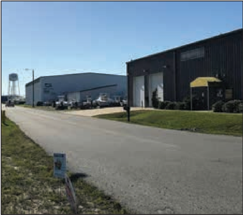
Warehouse structures in the Wanchese Marine Industrial Park
