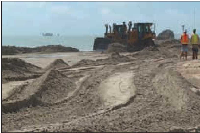
Beach nourishment work in Buxton
