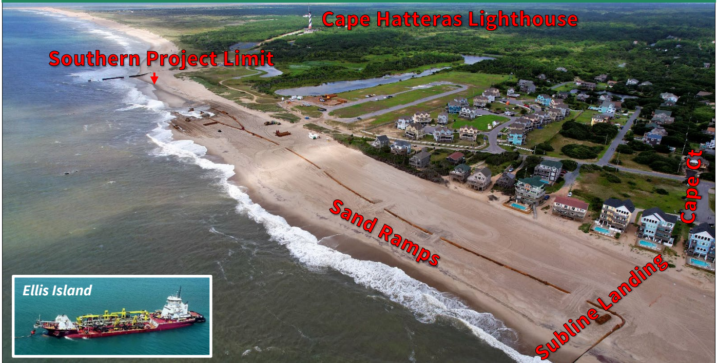
Pumping approaching the southernmost project boundary on Monday morning, July 11, 2022.
