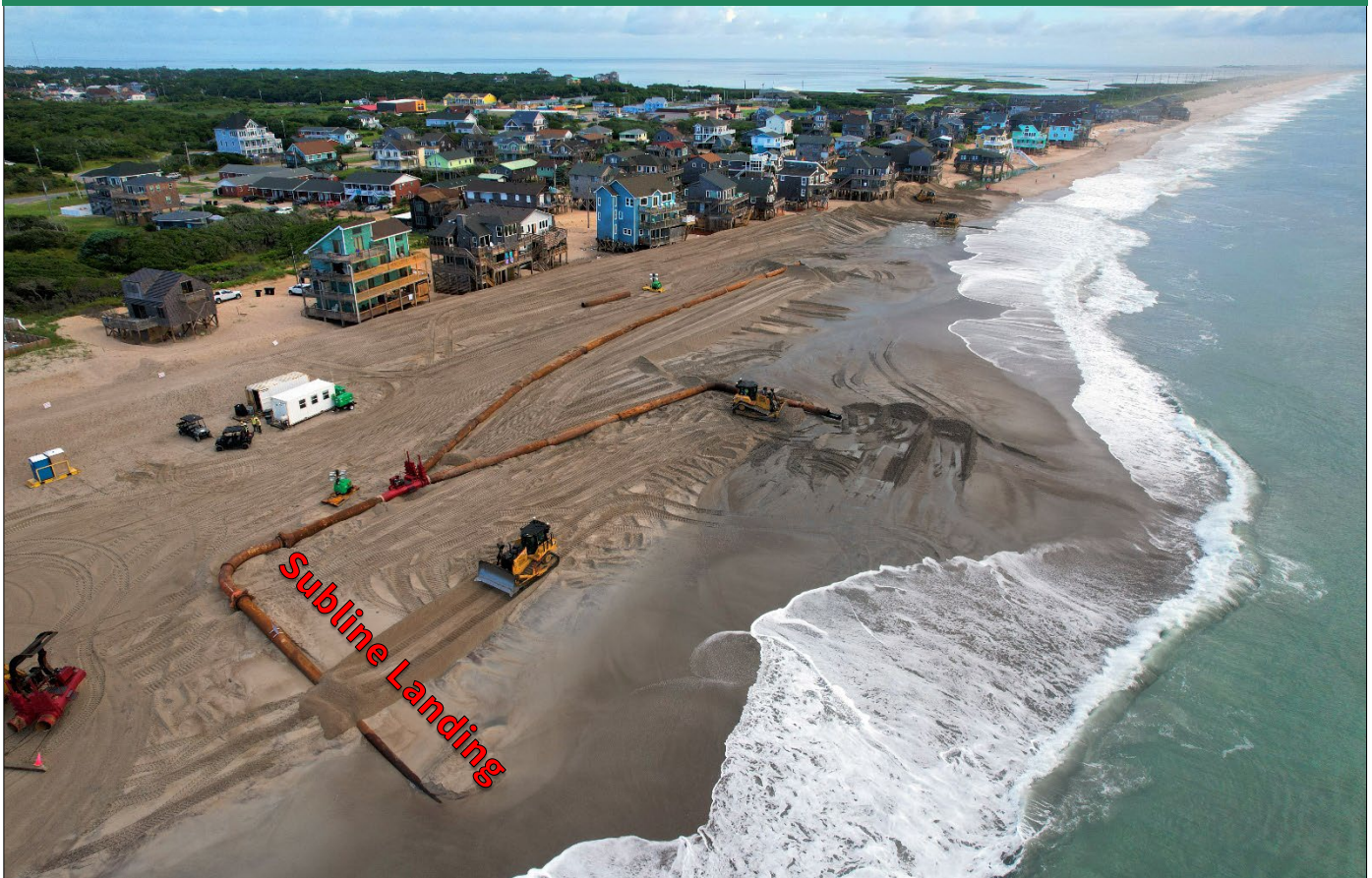
Construction started proceeding north toward the National Seashore. [Photo July 12, 2022]
